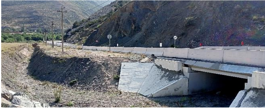
Figure 2. Dry channel near the tailings dump.
